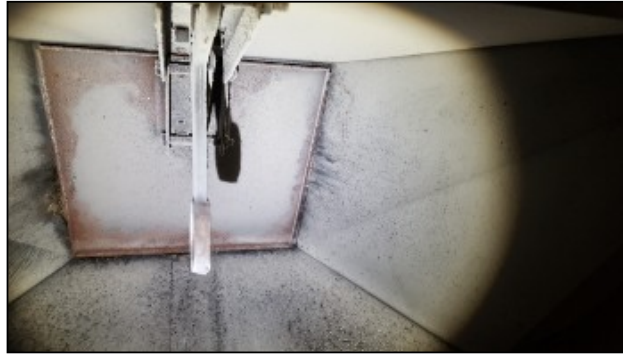
No clamp installed
