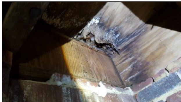
deterioration under fireplace
