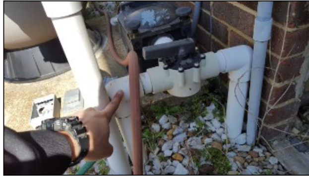
turns off bottom drain
