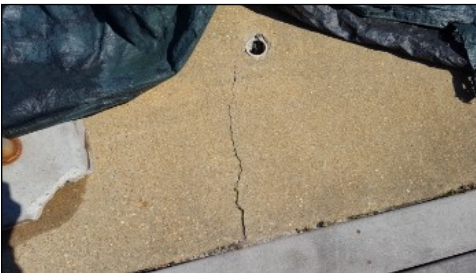
crack at ladder anchor
