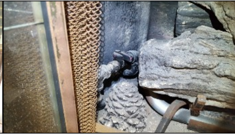
gas valve is shut off
