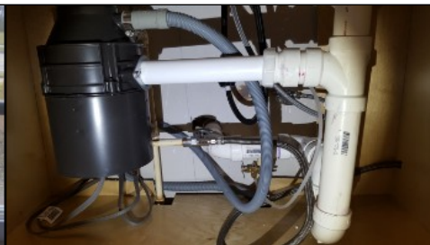
Missing high loop
