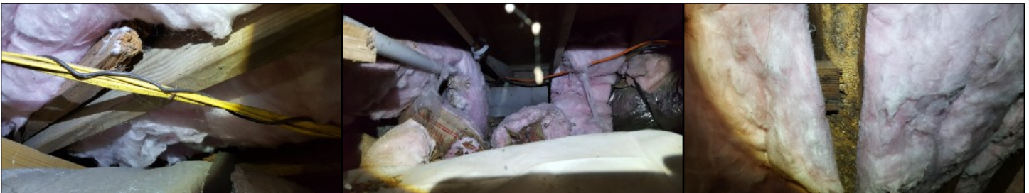
Previous WDO damage
