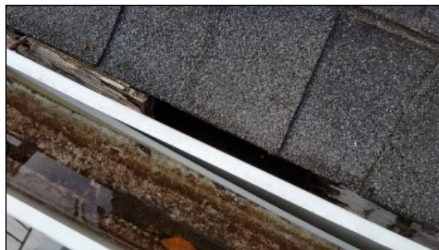
Wood deterioration
