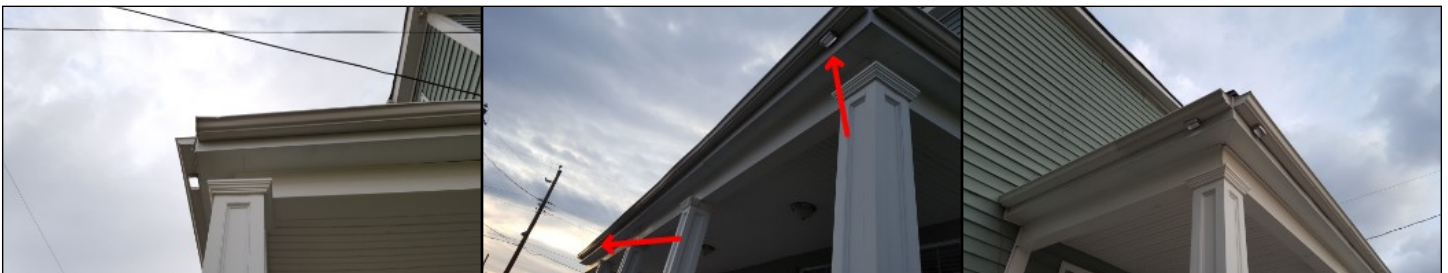
leaking gutter cap
