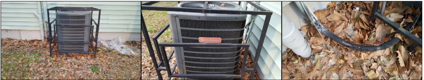
insulation deteriorating
