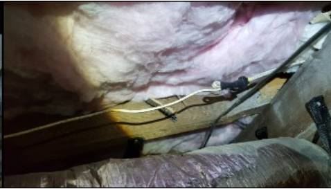
Splices should be done in a junction box
