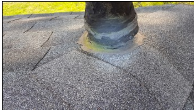
cracking caulk
