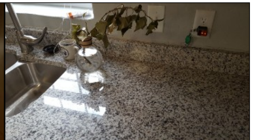
Not GFCI protected
