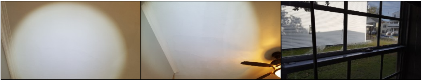
Previous repair in living room
